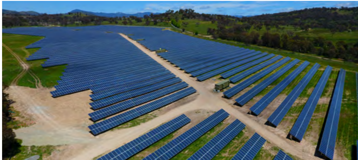
MUGGA LANE SOLAR FARM, AUSTRALIA 15.2 MWp, 2016
